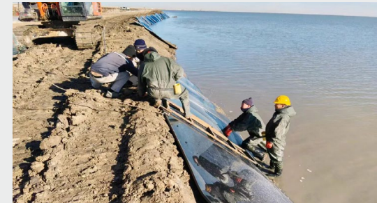
On-site Work to Ensure Production Safety During the Flood Season
