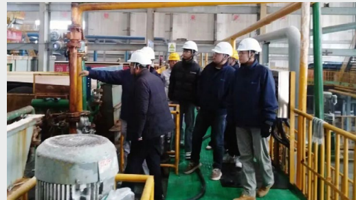
External Safety Technology Consultant Providing Inspection and Guidance
